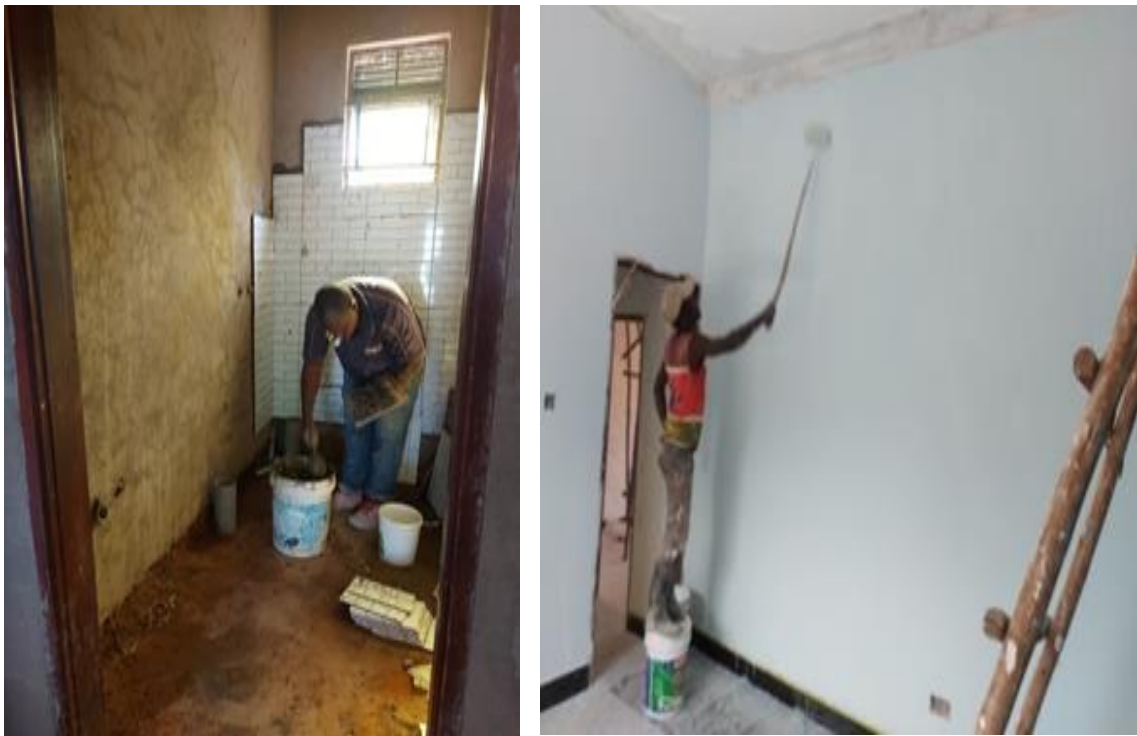
Figure 37: Construction and House Renovation
